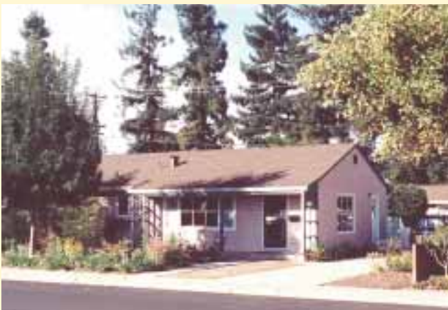
The large PV array on this cute little home is almost invisible from the street.
