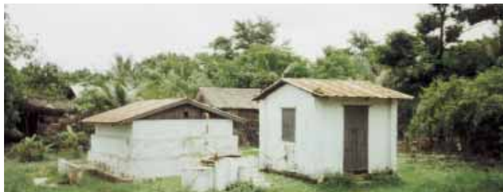
A large slow sand filter (structure on left) in a village in Myanmar.
