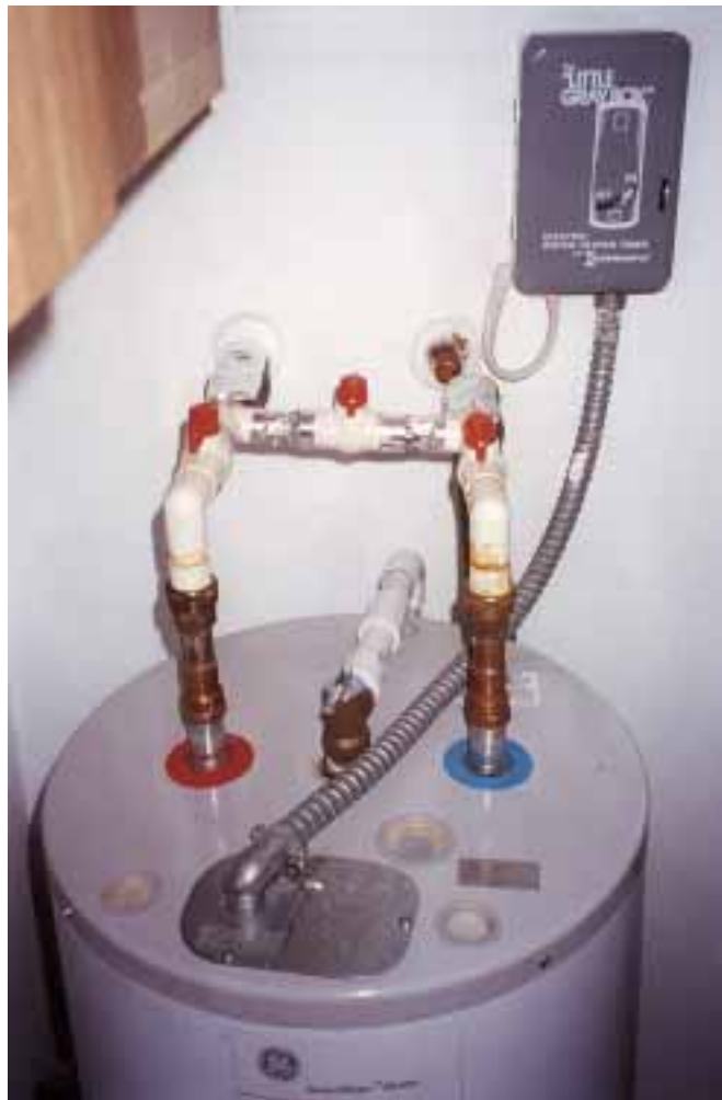
On the electric water heater, the timer switch and bypass valves are arranged for easy access.
