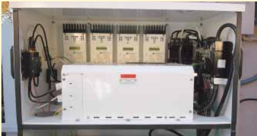
The top bay of the Trace Power Module, including the SW5548 inverter and four, C40 charge controllers (one is a spare).
