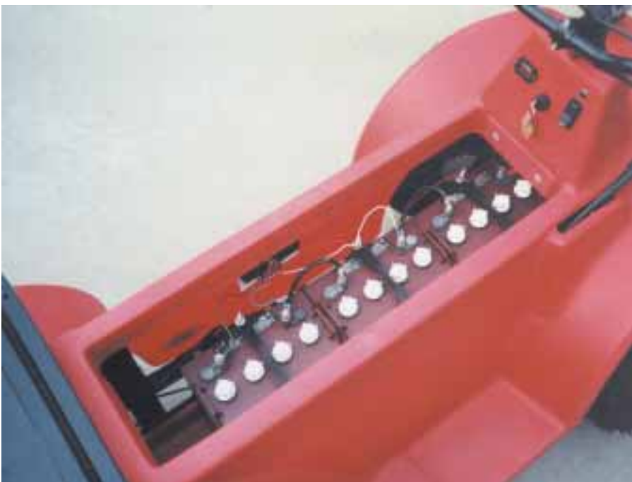
Under the hood—the gorilla's battery bank.
