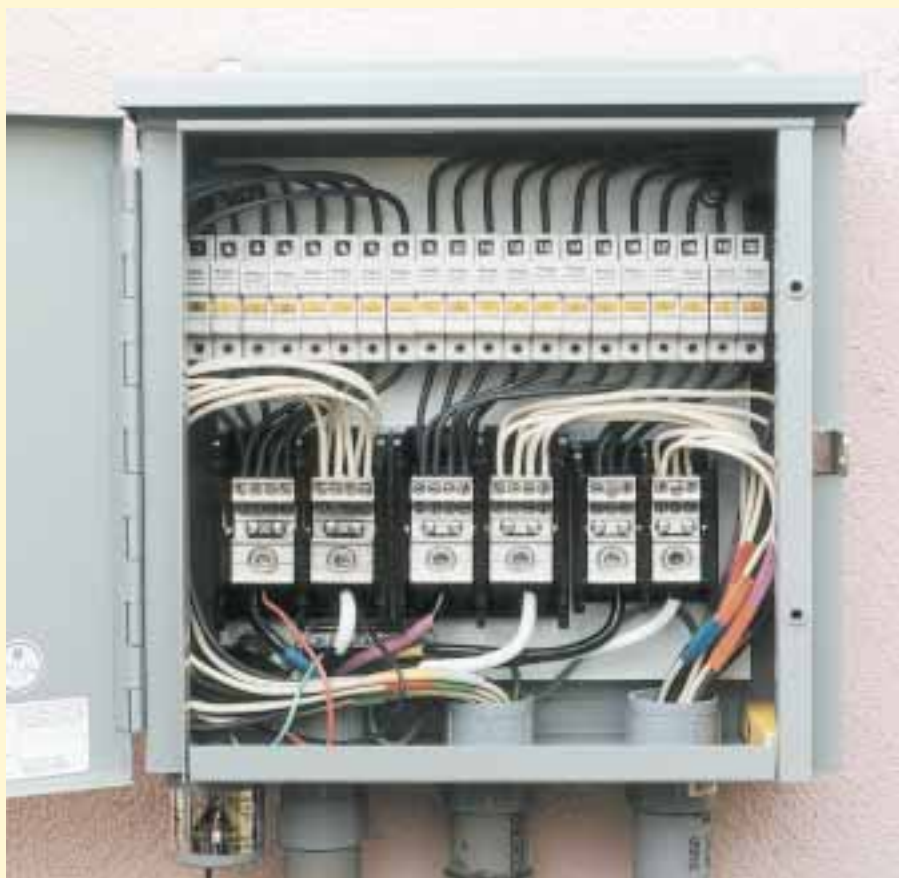
The PV combiner box brings together twenty, 48 volt subarrays, each consisting of two, 24 volt modules.
