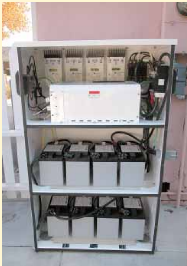
The Trace Power Module holds system components, including batteries, in a weathertight enclosure.
