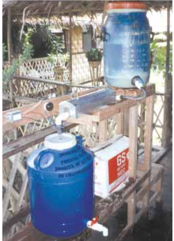
An 8 watt UV purifier with a 12 V, 100 AH battery (in box) and a slow sand filter (top barrel), in an MSF clinic.
