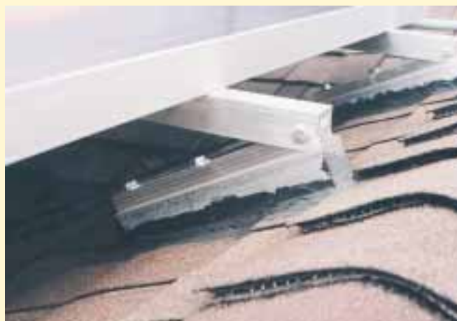
The upper mounting brackets are along the roof ridge.
