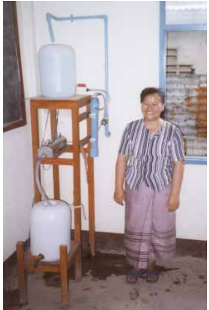
A slow sand filter, cloth filter (blue tube), and 8 watt UV purifier at a secondary school in Vientiane, Laos.
