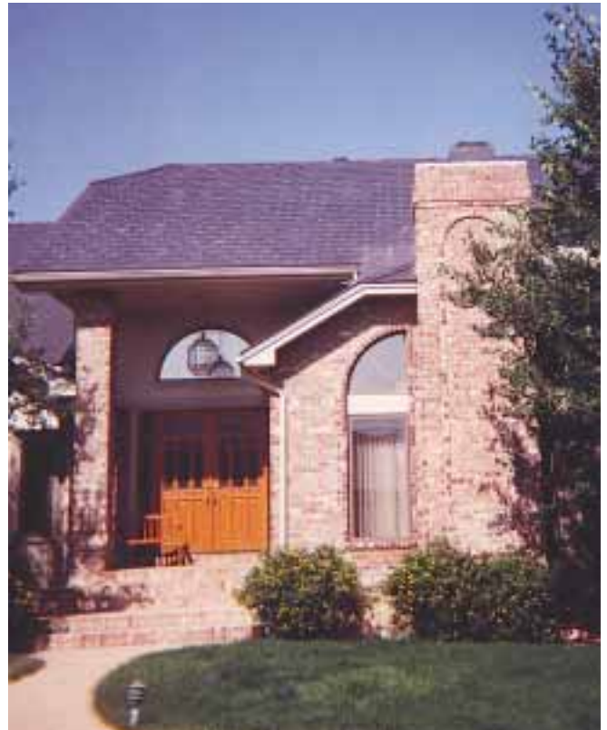
The SunSlate PVs are hard to spot because they're also roofing material. They were installed here with a westerly orientation—which makes sense for some utility-interactive systems.
