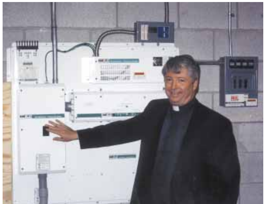
The power room is set up for demonstrations, and has been visited by bus loads of high school students.
